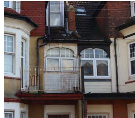
An example of poorly maintained balconies, the one on the right has been lost entirely
